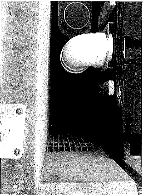
Old Containment Wall
