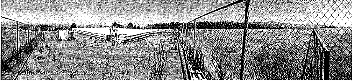
Photograph #11: Panorama of Facility from Northeast Corner
