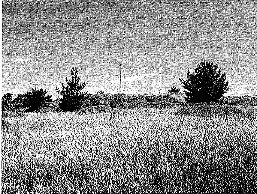
Photograph #5: Existing Power Utilities Adjacent to Tank Site
