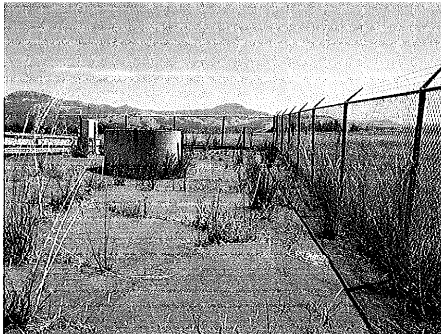
Photograph #10: Existing Tank Storage Facility, from Southwest Corner Looking North
