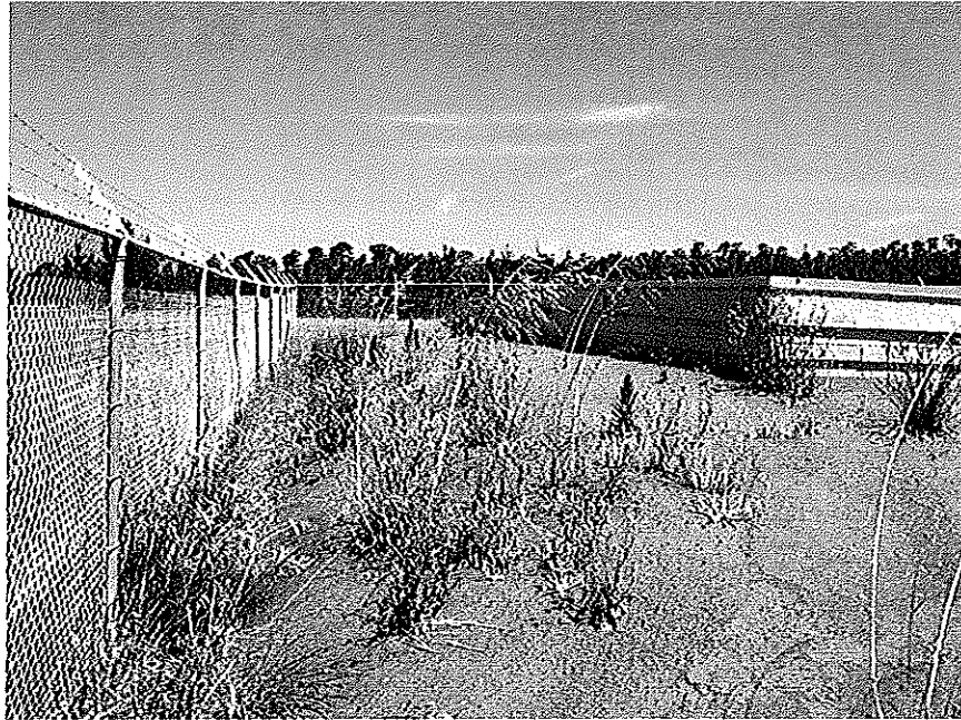
Photograph #9: Existing Tank Storage Facility, from Southwest Corner Looking West
