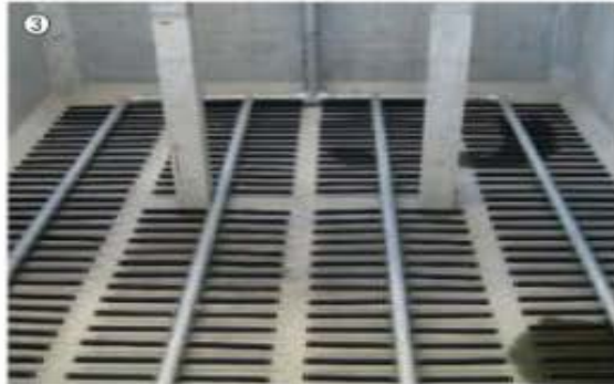
MBR bio-tank with fine bubble aeration individually calculated for the project
