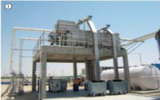
Mechanical pre-screening with 3 mm perforated plate or 1 mm bar spacing plus grit/grease trap
