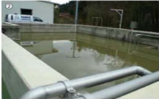
Buffer tank for a regular flow even with hydraulic peaks and varying loads, with simple aeration or with stirrer
