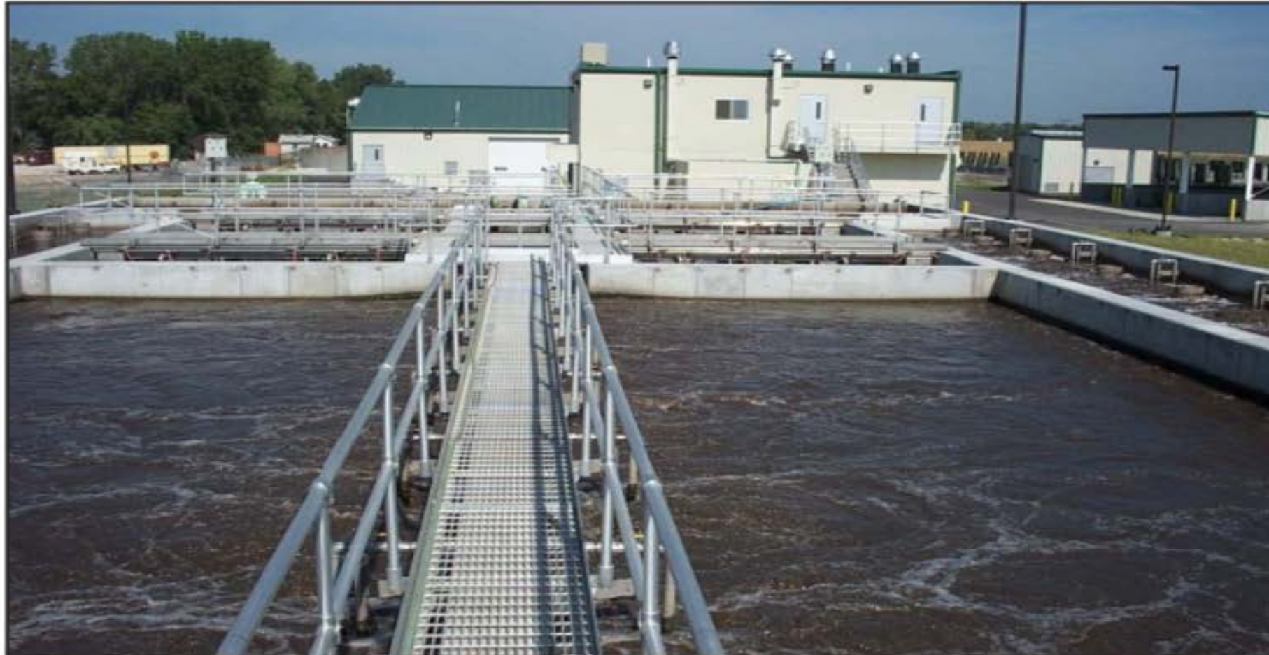
The rectangular layout of the SEQUOX Process results in a smaller footprint and easy expansion.
