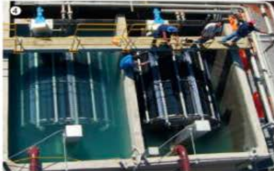
Huber VRM® filtration unit, 0.038 µm pore size, retaining bacteria, viruses and germs, wastewater diffusion through pump-generated underpressure
