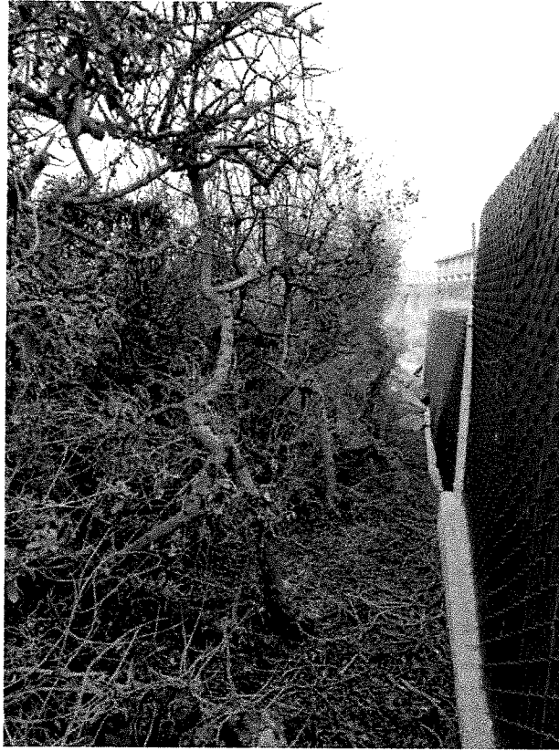
1 Non-native vegetation encroaching into WWTP
