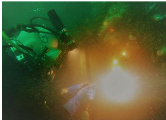
Figure 2: HOI Diver Burning Sheet Wall
