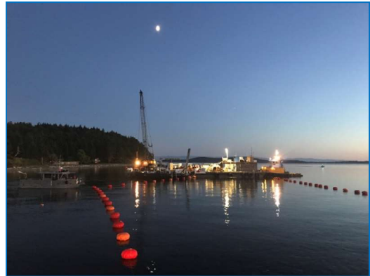
Figure 1: HOI Submarine Cable Installation
