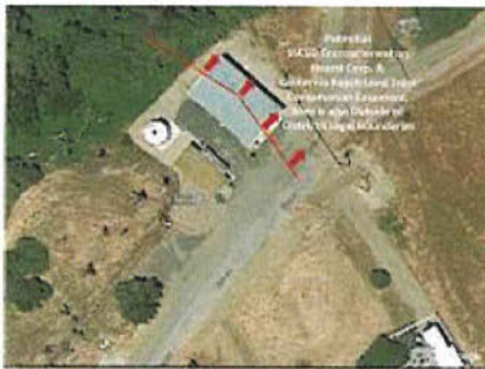
RO Building Potential Encroachment.jpg 167K
