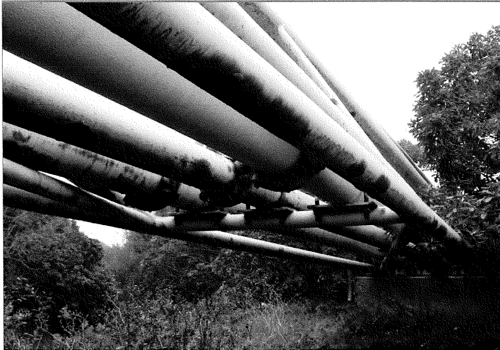
This view shows the typical condition of the bridge overall.
